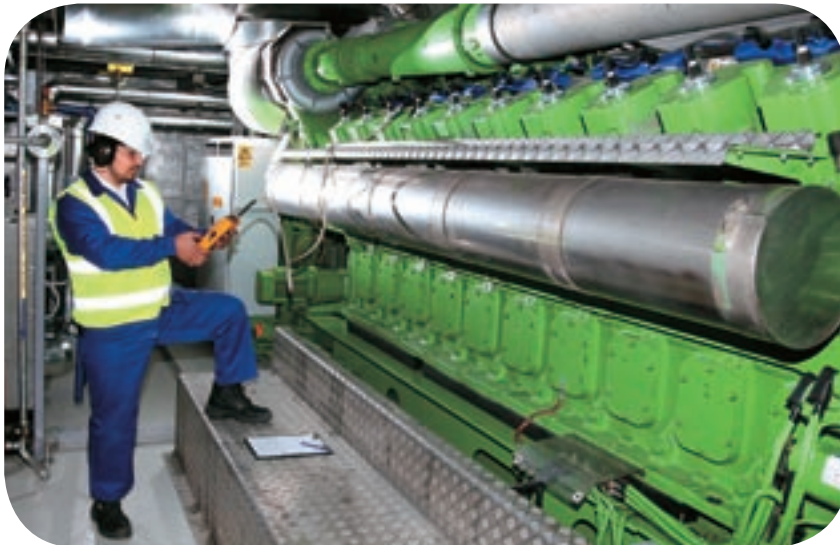
An engineer checks one of the Jenbacher engines at the CHP plant in Ploesti which opened in 2009.
